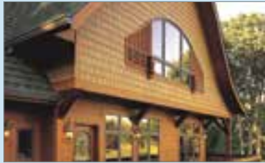
Fiber Cement Siding
