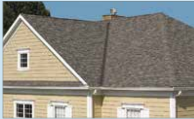
Roofing and Ventilation
