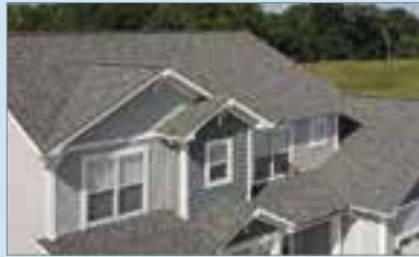
Roofing and Ventilation
