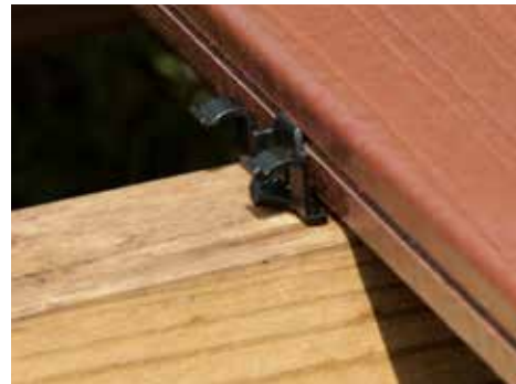
The clip is installed into the groove; then, a screw is driven into the joist at an angle.
