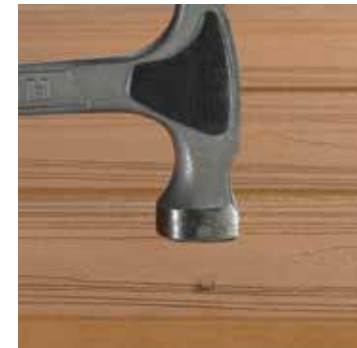
A color-matched plug is tapped in with a hammer.
